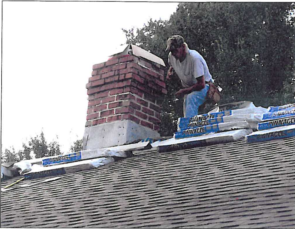
Chimney flashing repair.
