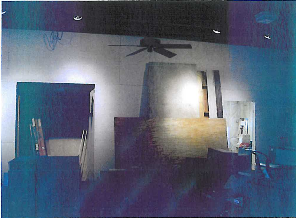
Photograph P7 – New partition in Freight Room creating accessible restrooms and a small office space for the proposed multipurpose facility. Note recently installed general and display lighting and ceiling fans.
