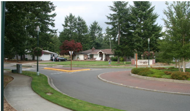
Photo 5-1, Single Lane Roundabout
