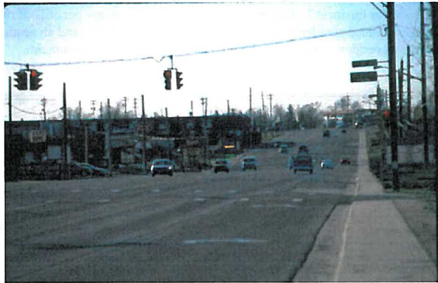
South Golden Road before Improvements
