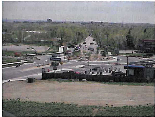
South Golden Road/Ulysses Street Roundabout
