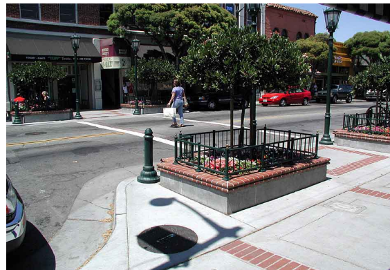
Figure 15 - Special lighting and landscape treatments highlight crosswalks for pedestrians and motorists. Similar treatments may be used to announce special districts or downtown areas.
